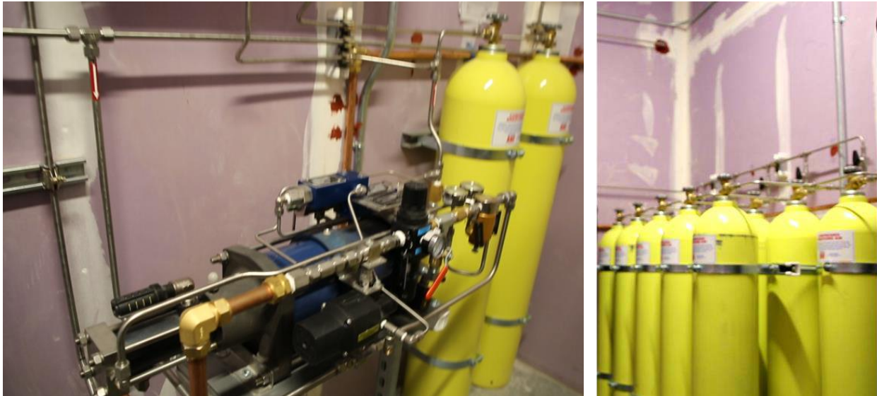
(a) Primary storage with booster pump
