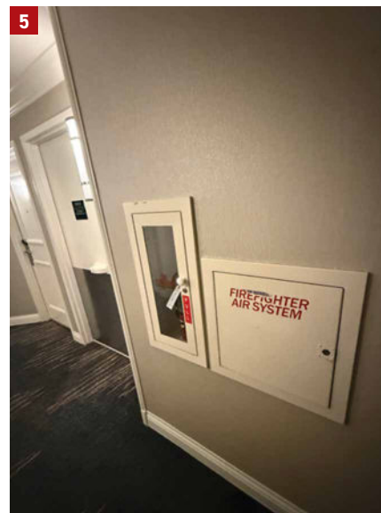
5. Integrating solutions such as FARS gives responders the ability to extend working time, rotate crews effectively, and maintain operations without retreating to ground level.
