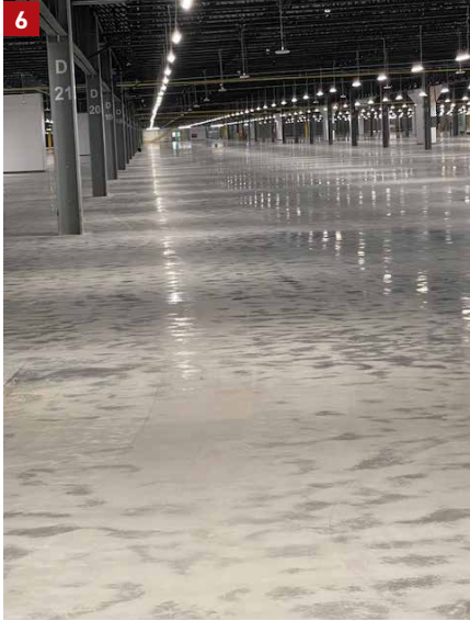
6. The column closest to the camera is marked D-21. There are at least 20 additional bays between the columns. If you haven't adequately planned before the fire, it will be way too late to do it during the fire. (Photo by John Feehan.)
